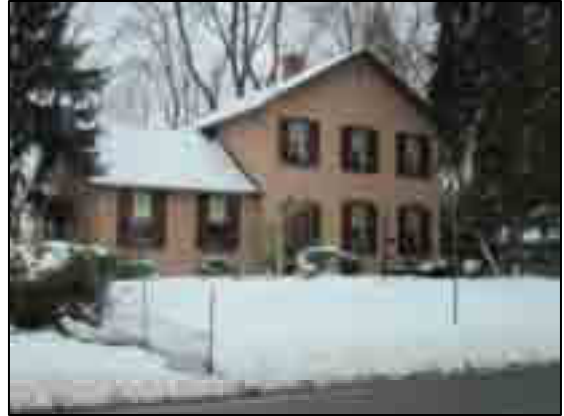
This mid nineteenth-century home has a new side wing. The wing matches the window size and other details of the original house. The main block with side wing massing is typical of mid nineteenth-century vernacular homes.
