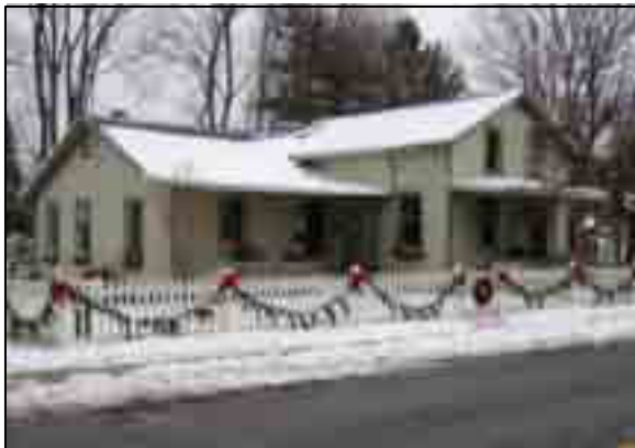
The wing added to this early nineteenth-century home matches the window design and spacing, porch details, and roof form of the original house.
